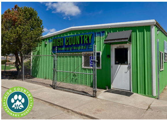
EXISTING VETERINARY FACILITY 1,861 SF | Seller Leaseback
