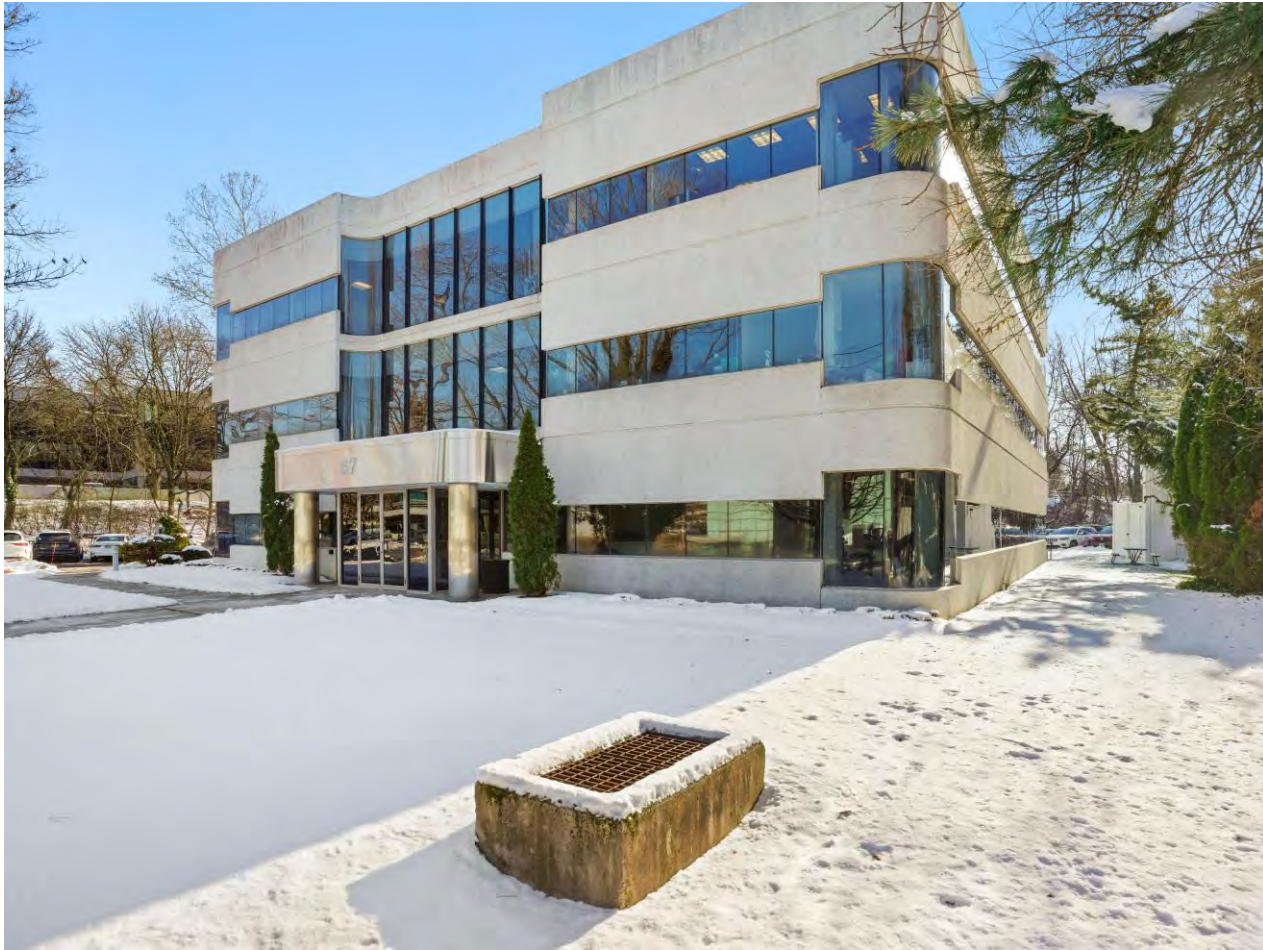
Exterior of Building
