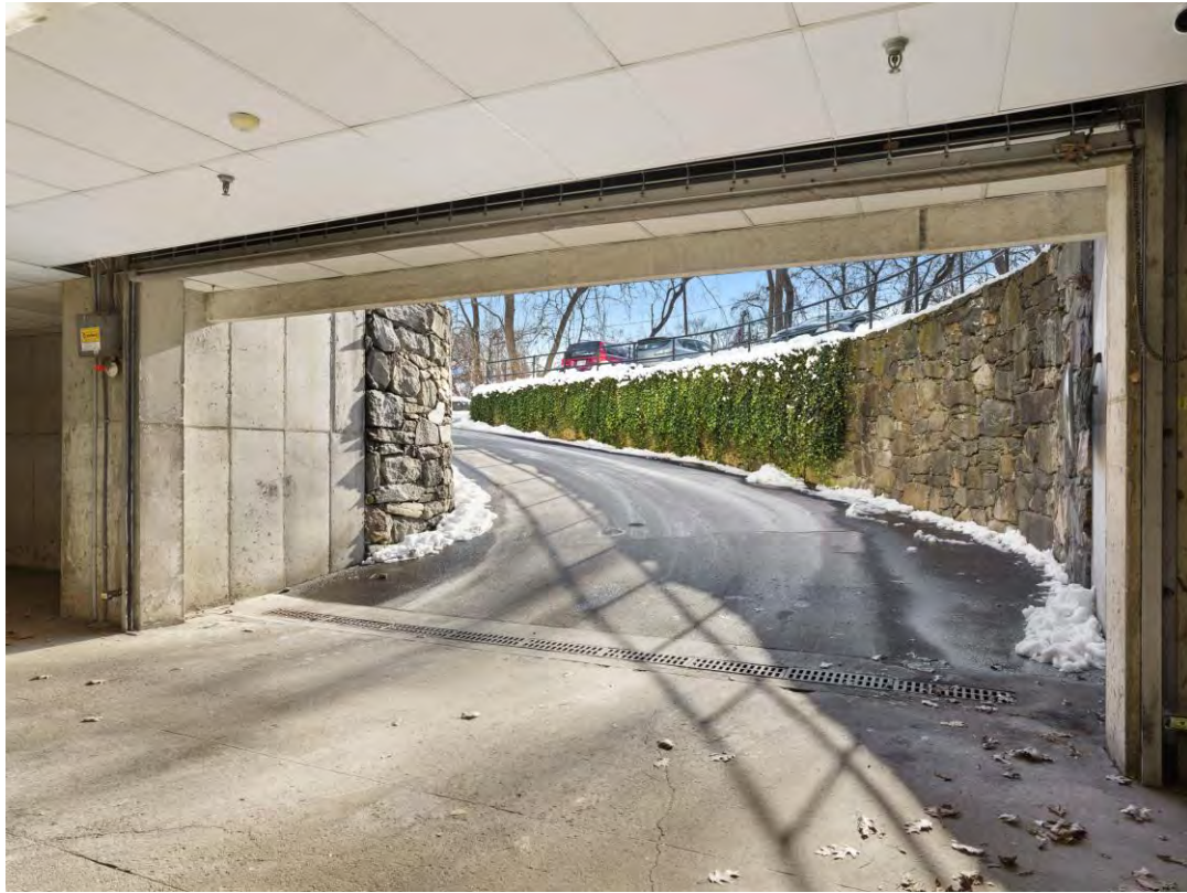
Indoor Underground Garage Entrance
