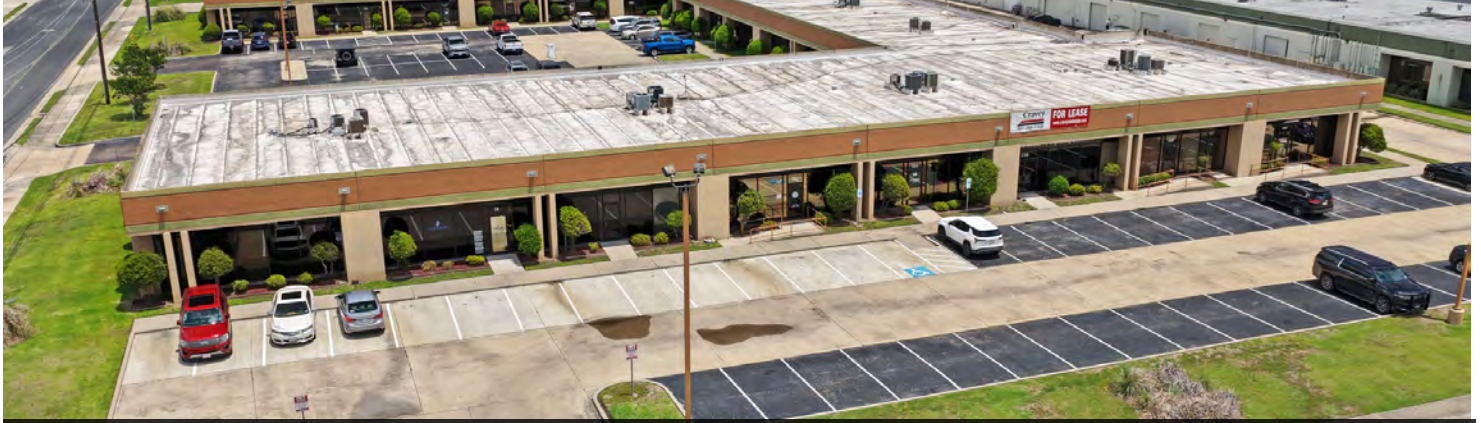
Traditional office suites fronting S. Enterprize Parkway are served by a shared west-side parking area offering approximately 50 parking spaces.
