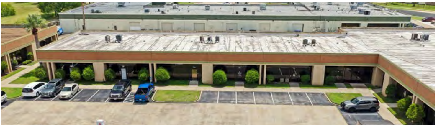
The flex office/warehouse suites are centered around a spacious interior parking court in a horse-shoe configuration offering approximately 76 parking spaces.
