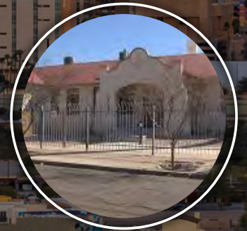
CONSTRUCTION BEGINS ON DUNBAR PAVILION BUSINESS EMPOWERMENT CENTER
