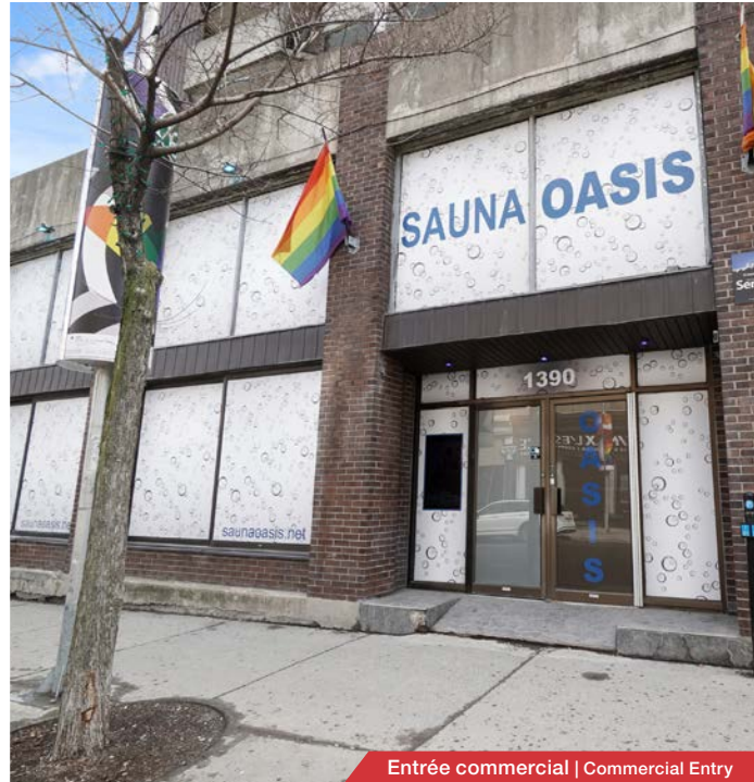
Entrée commercial | Commercial Entry
