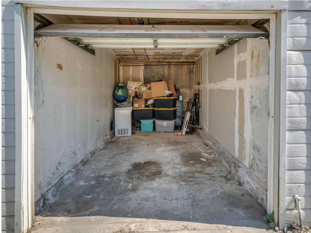
2161 Locust Ave Inside Garage
