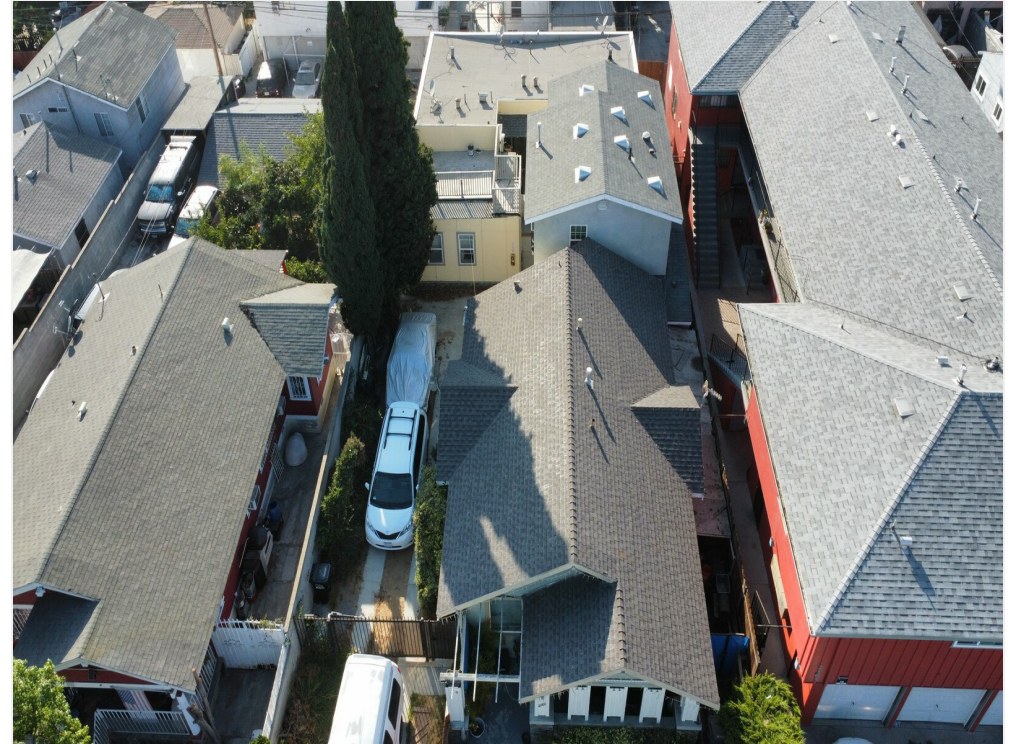
2161 Locust Aerial Back Units
