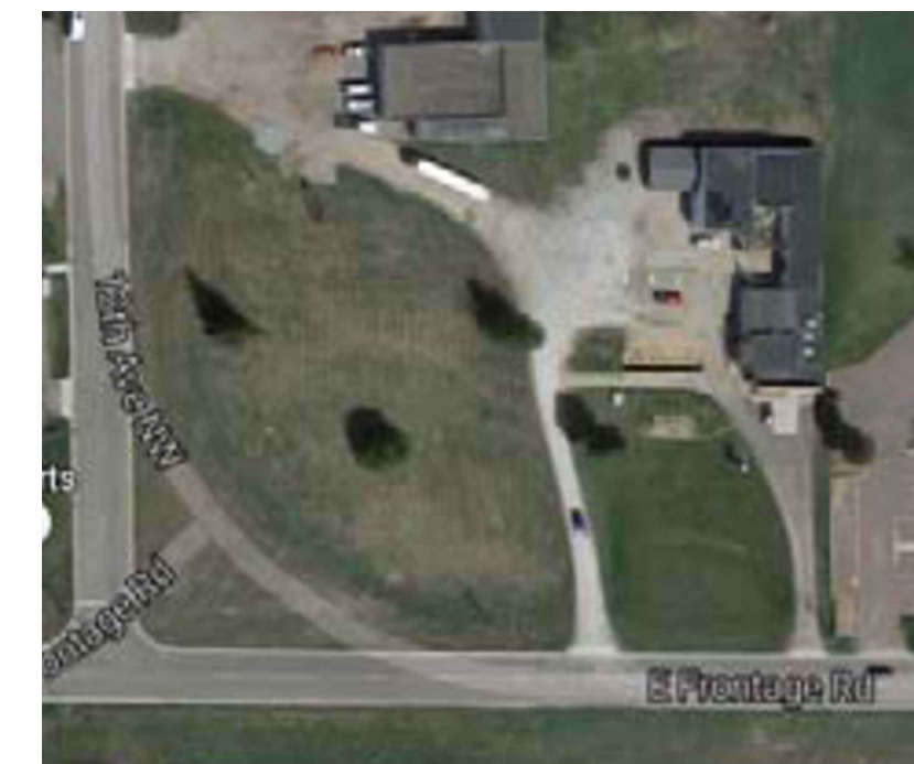
AERIAL PHOTOGRAPHY NOT TO SCALE (Photo from Google Maps)
