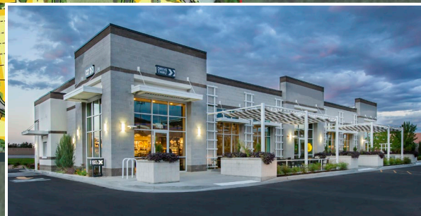
RETAIL/COMMERCIAL SPACE GAS/C-STORE | RETAIL | OFFICE | HOTEL RESTAURANTS | QSR/FAST FOOD
