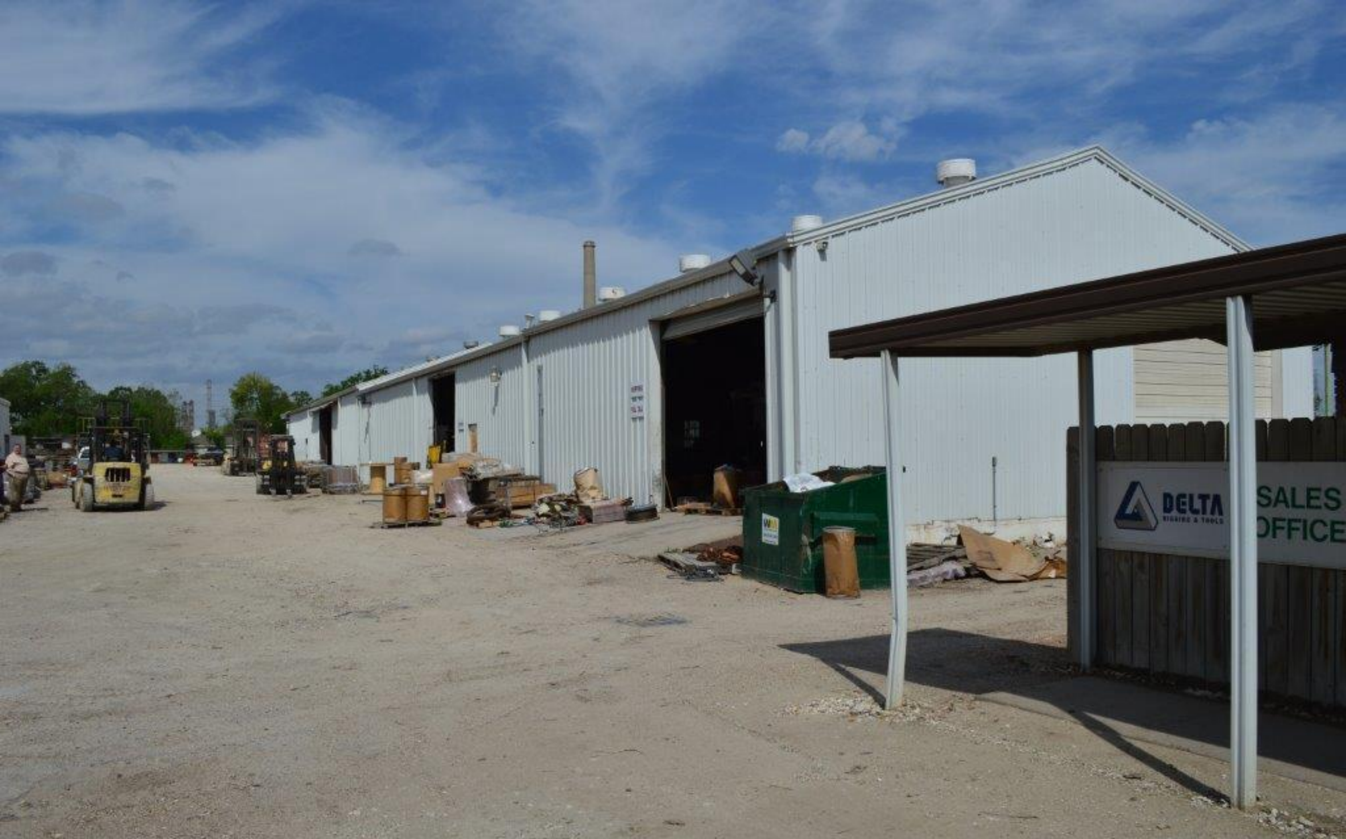
View of 9,000 sf warehouse from rear of Office Building
