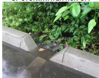
PARKING LOT ISLAND: SUSTAINABLE DESIGN OF RAISED CURB FOR REUSE OF STORMWATER RUN-OFF
