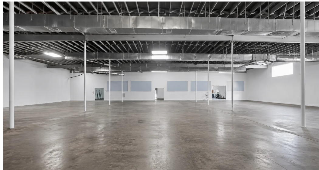
Fully Conditioned – 17' Height – 15' x 32' Column Spacing
