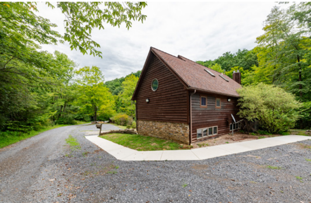
Main House (Building 1)
