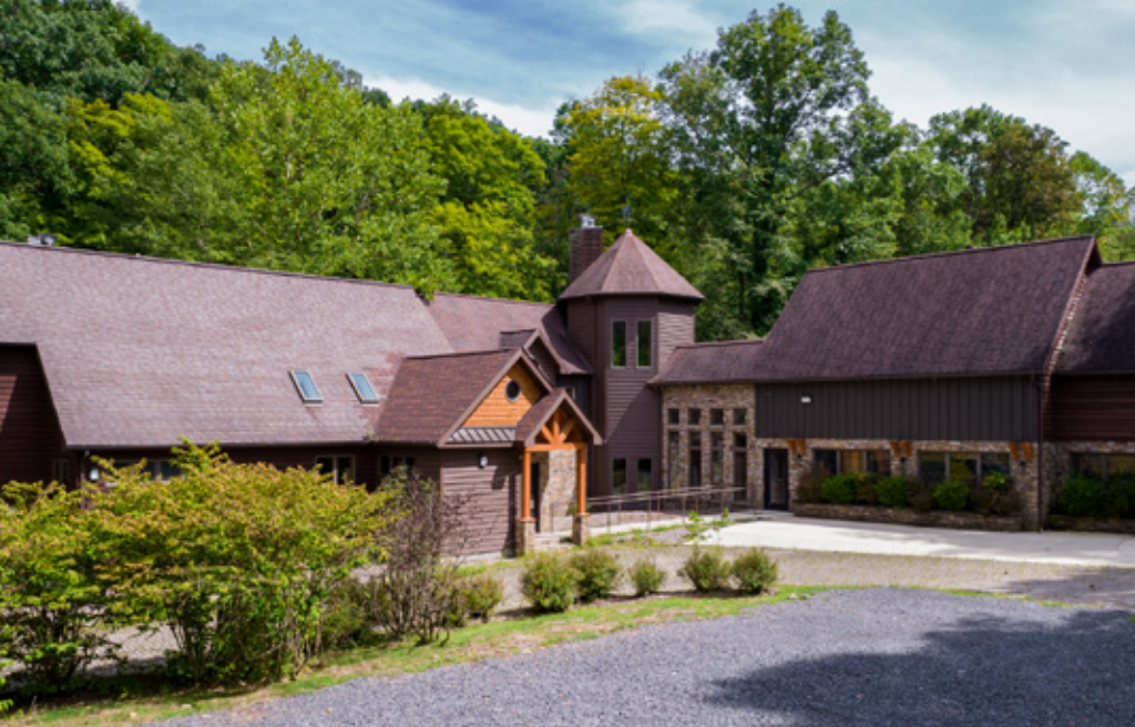
Main House (Building 1)
