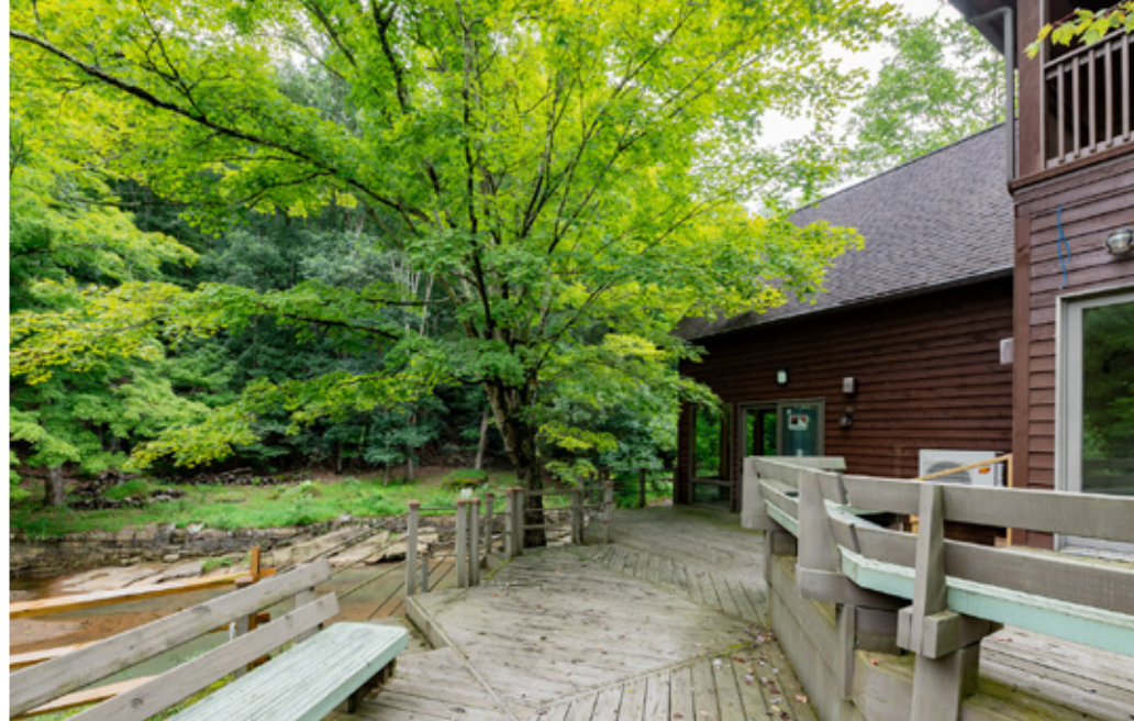
Main House (Building 1)
