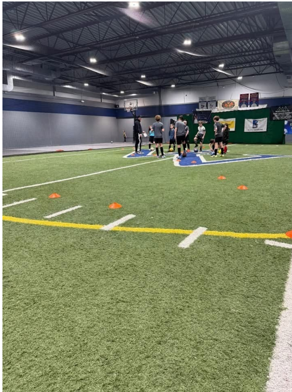
Clear-span floor supports active recreation & sport uses
