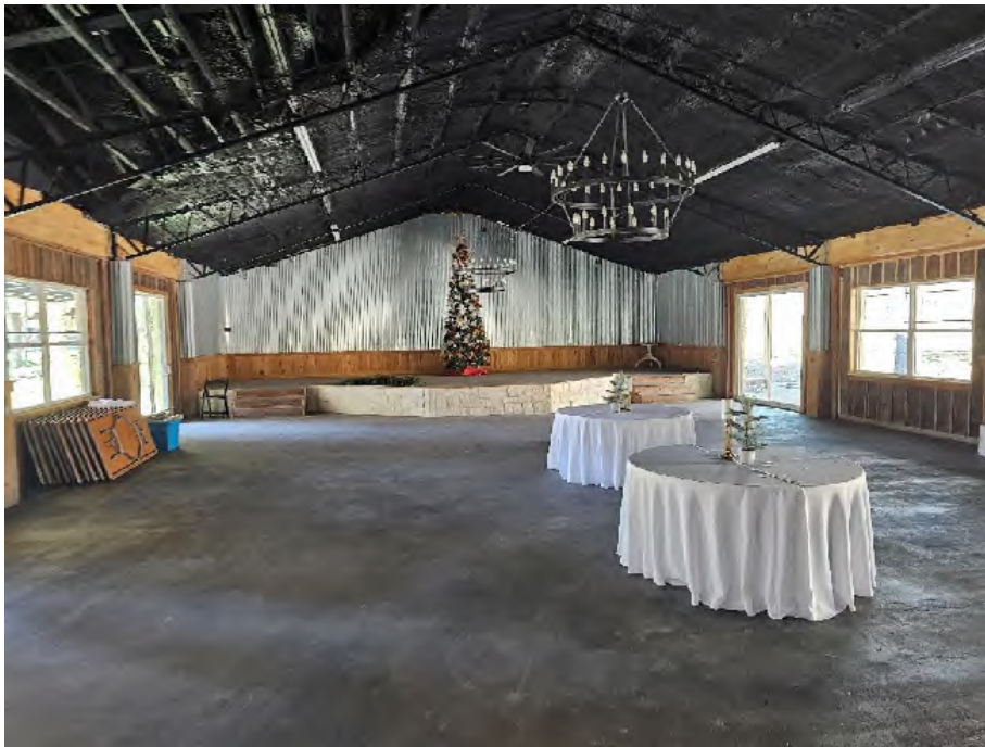
View of Event Center Interior
