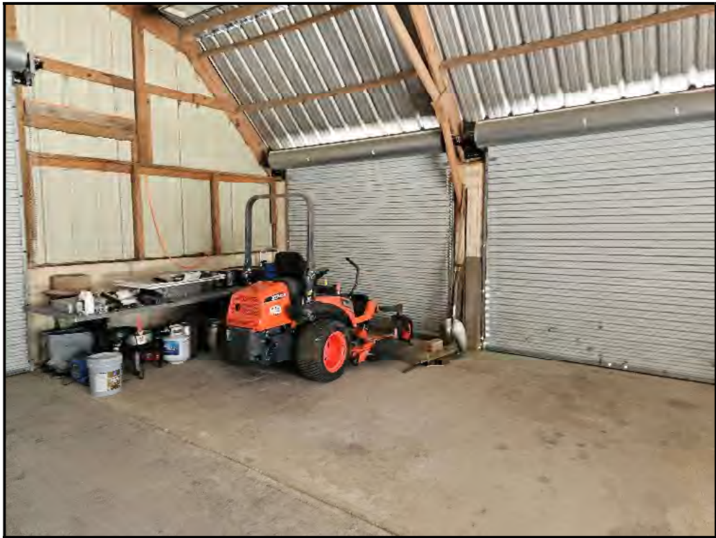
View of Interior of Barn
