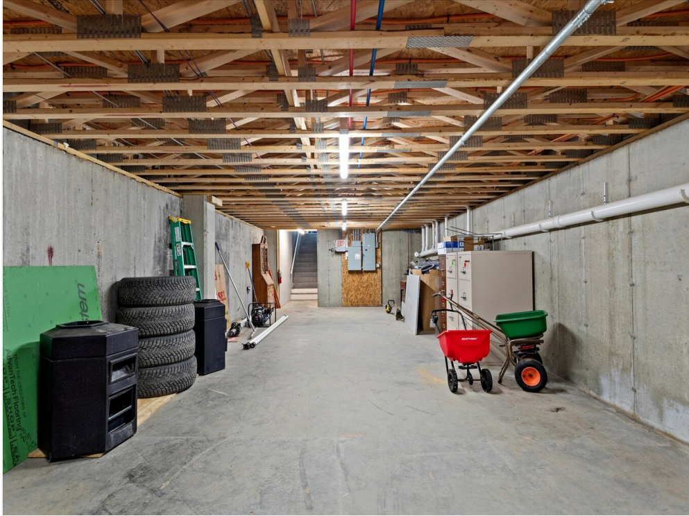
30-86 Parsons St, Basement
