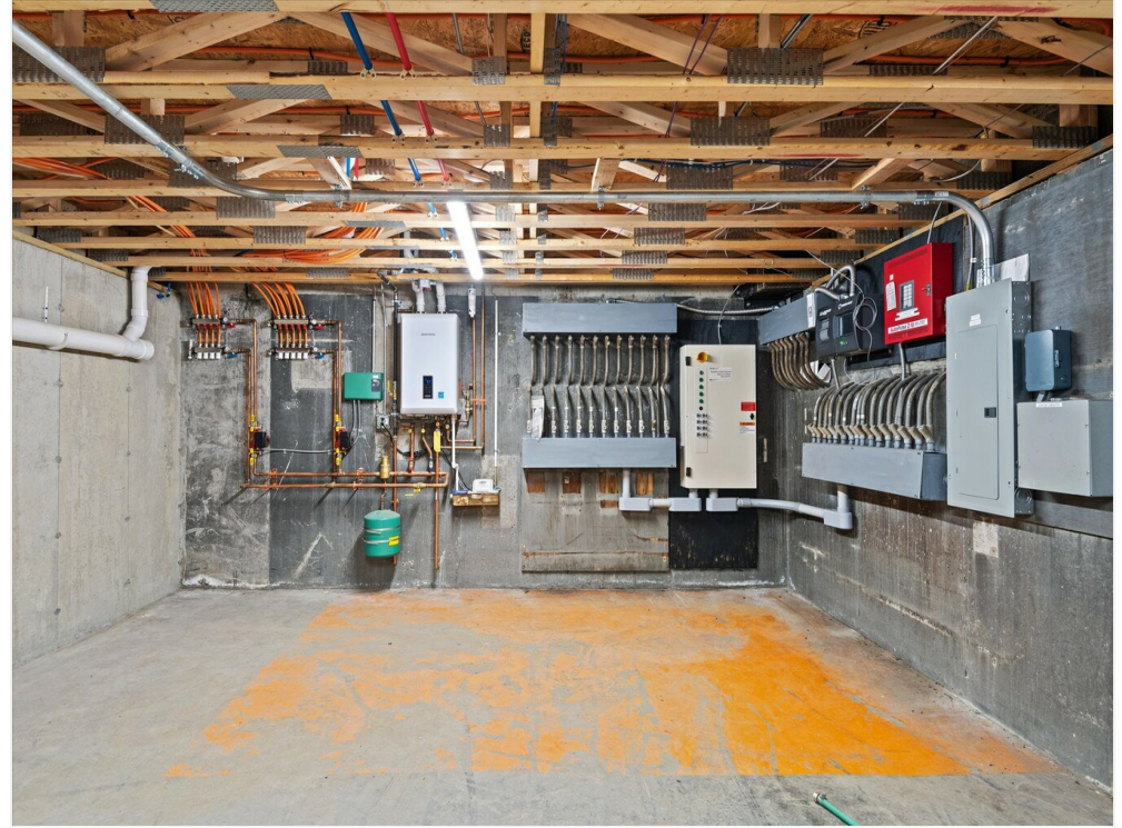
28-86 Parsons St, Basement
