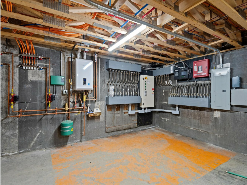
29-86 Parsons St, Basement
