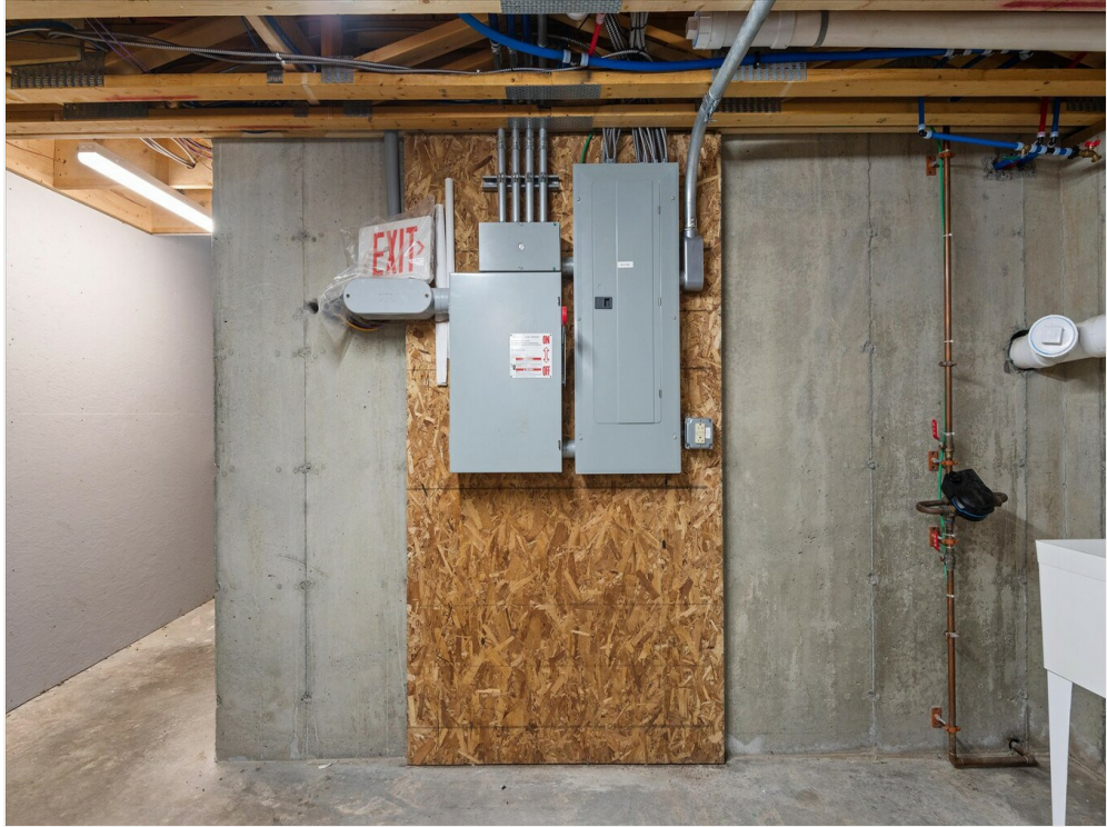
31-86 Parsons St, Basement
