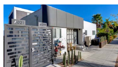
2 4017-21 Georgia St 14 units
