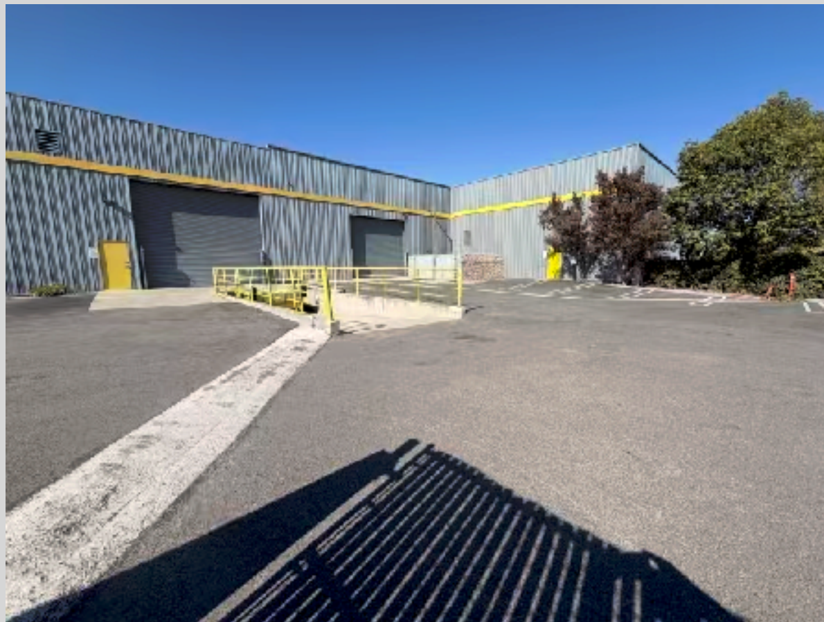
1 truck well and 1 grade-level door
