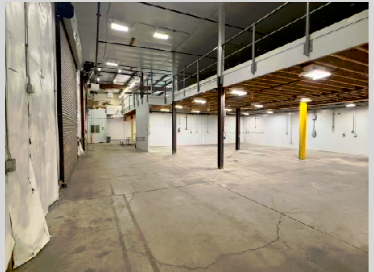
Mezzanine with fork-lift access
