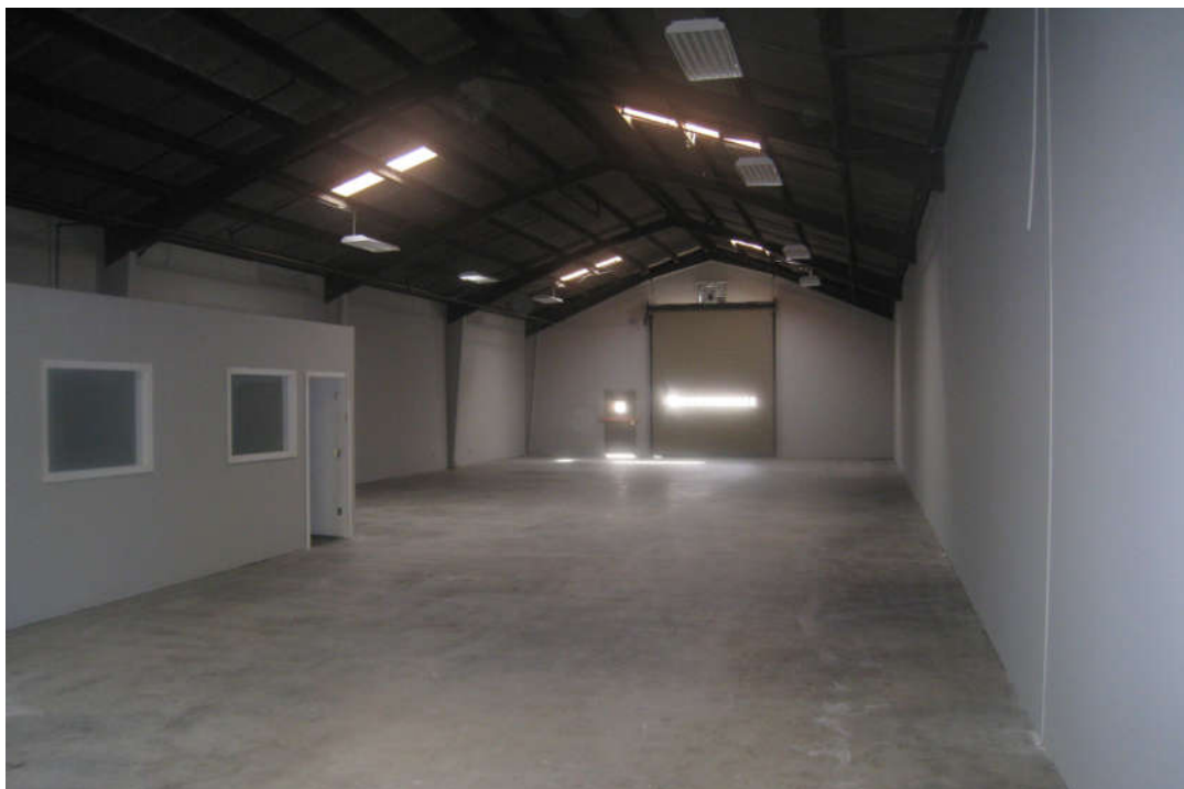
Fully Insulated and Sprinklered Warehouse
