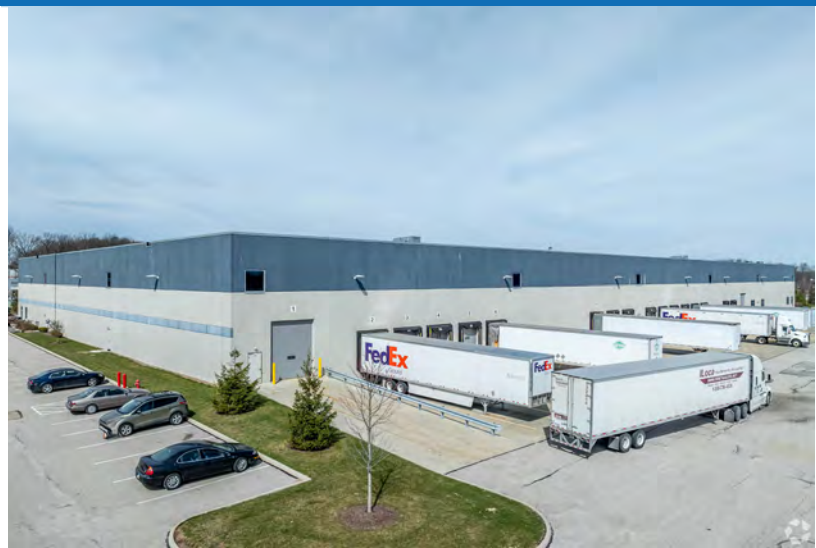
Exterior View: Drive-in Doors and Docks
