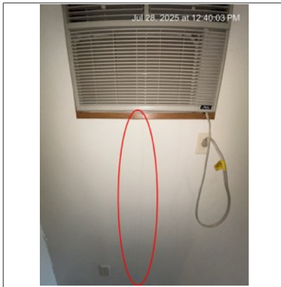
Moisture from AC condensation running down the wall - recommend repair to prevent deterioration of exterior wall.
