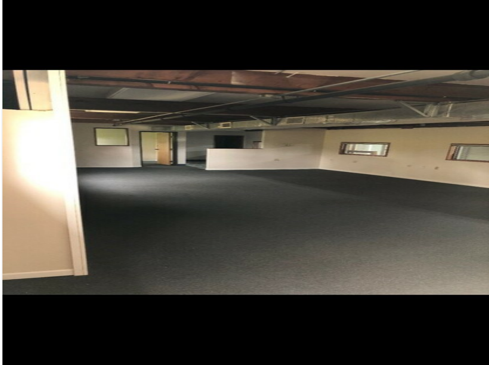
Fully Functional Second Level Office Space
