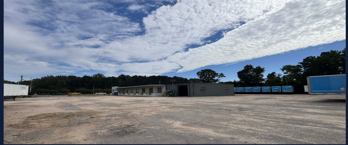
Exterior — Truck Court & Yard
