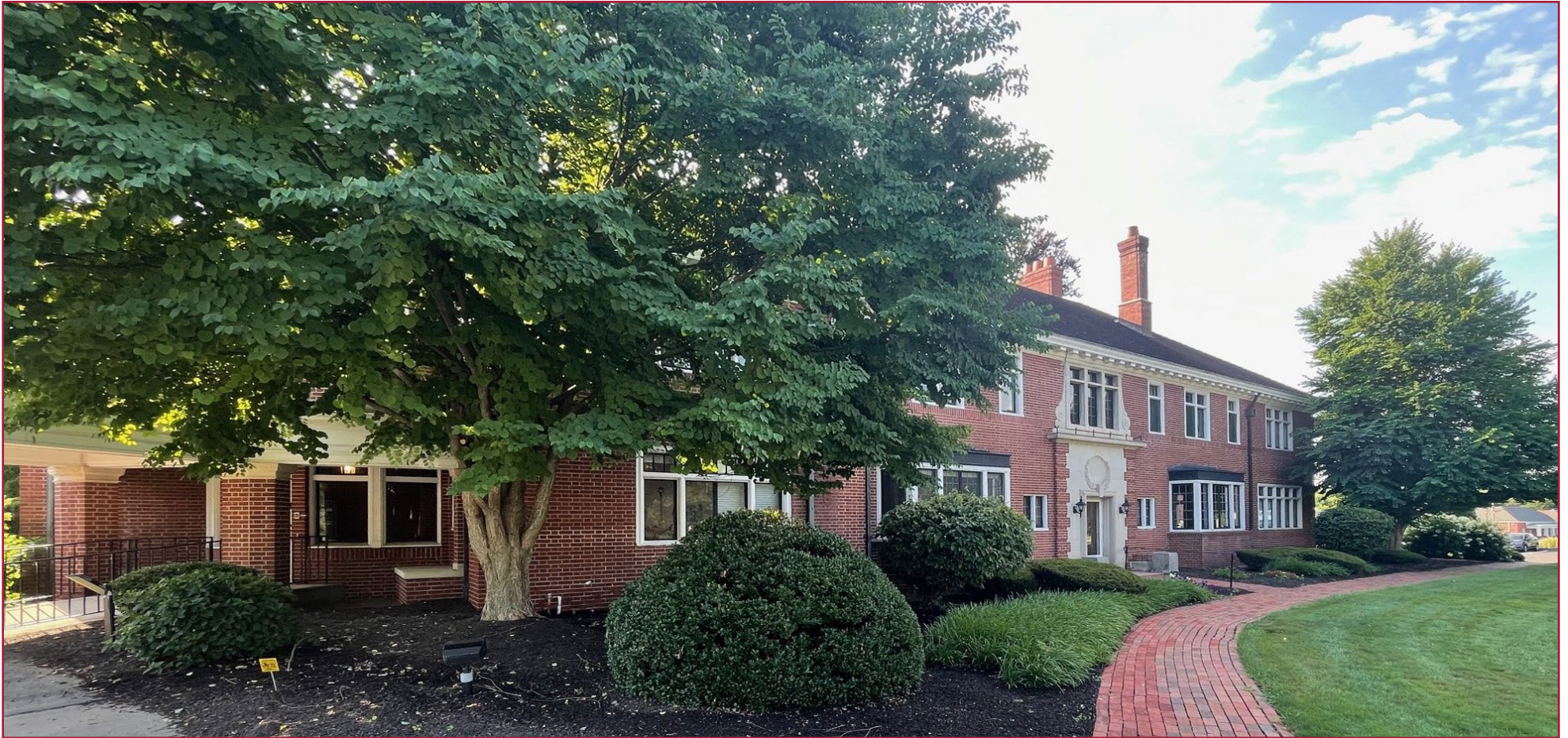
The Cannon Building is situated directly on State Routes 10 and 202 and offers the opportunity for retail uses, a conversion back to residential, or continued use as office space.
