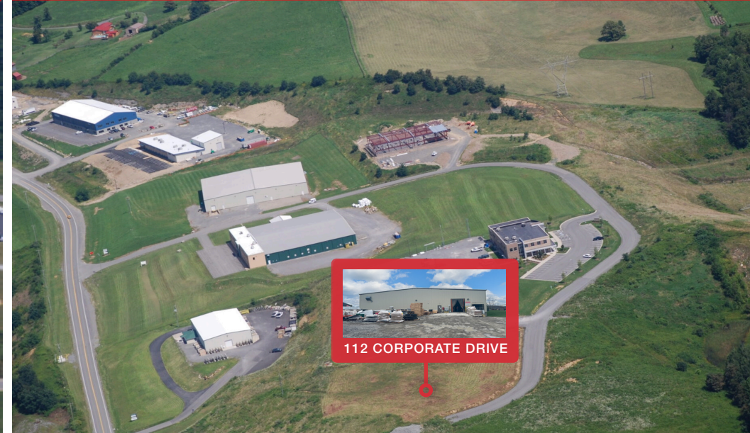
CHAPLIN HILL BUSINESS PARK AERIAL VIEW
