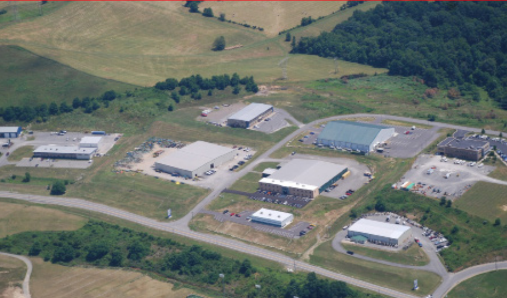
CHAPLIN HILL BUSINESS PARK AERIAL VIEW
