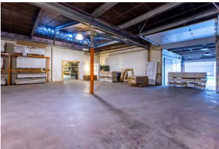
Enclosed loading dock
