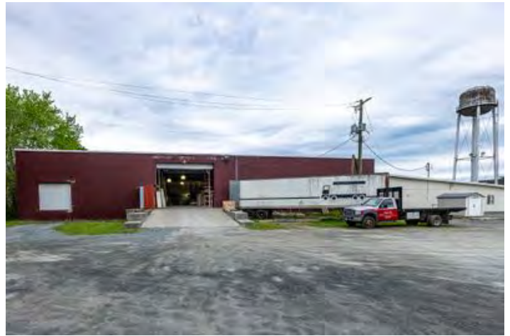
Rear ramped access
