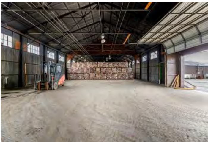
Lumber storage metal pole barn showing ramped access
