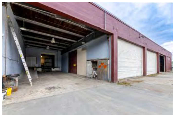
Enclosed loading dock
