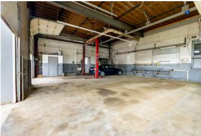
2 Bays of front mechanics garage
