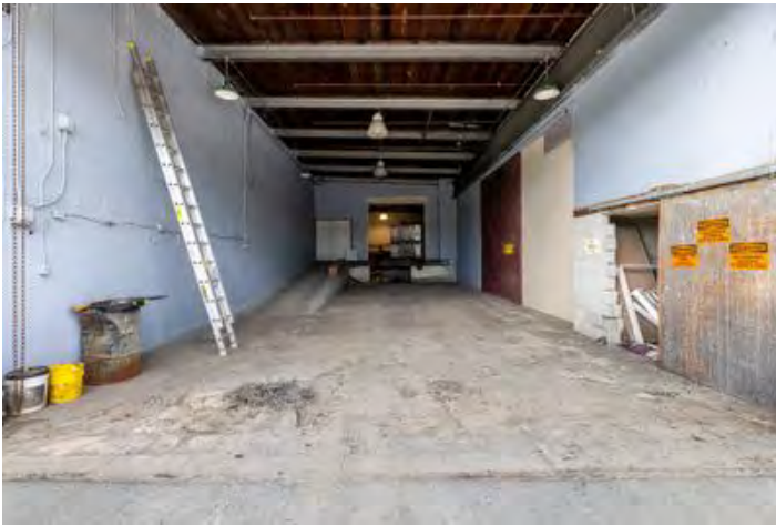
Enclosed loading dock
