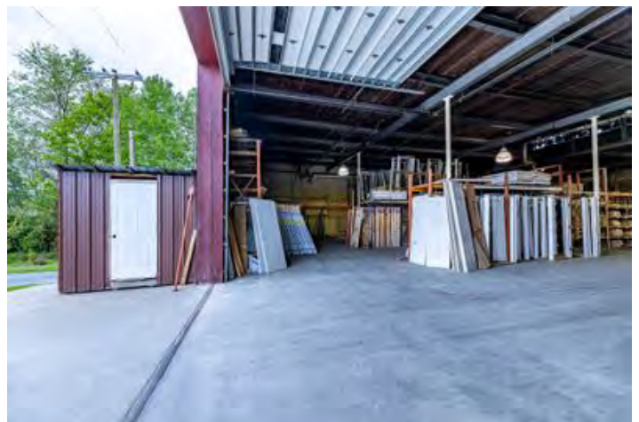
Rear ramped access
