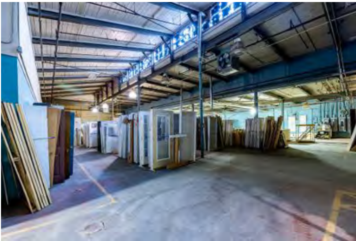
Portion of warehouse showing clerestory roof windows
