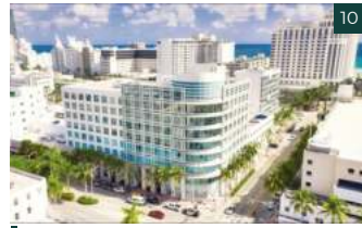
10 BLACK LION + MASSA | 1601 WASHINGTON AVE 8-STORY OFFICE CONVERSION WITH LARGE HOSPITALITY VENUE
