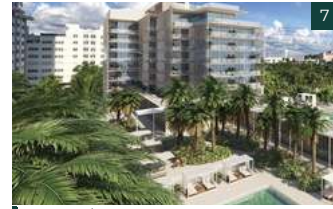
7 BVLGARI HOTEL | 100 21ST STREET 100-KEY HOTEL WITH A SPA AND RESTAURANT/BAR FROM CHEF NIKO ROMITO
