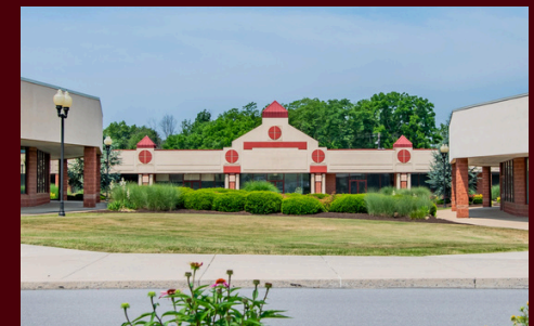
Center View of Outlet
