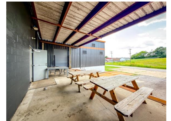
Covered Docks & OH Doors
