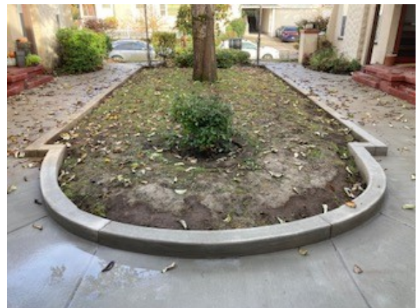
Courtyard Features All New Concrete
