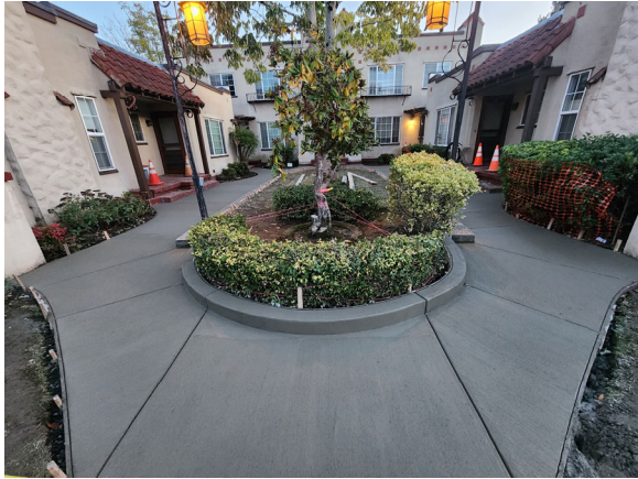
New Concrete Courtyard Walkway 2025
