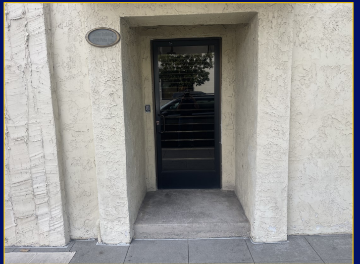
Main entry from Palm Avenue
