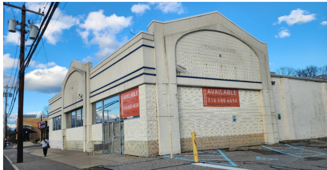
South Facing View
