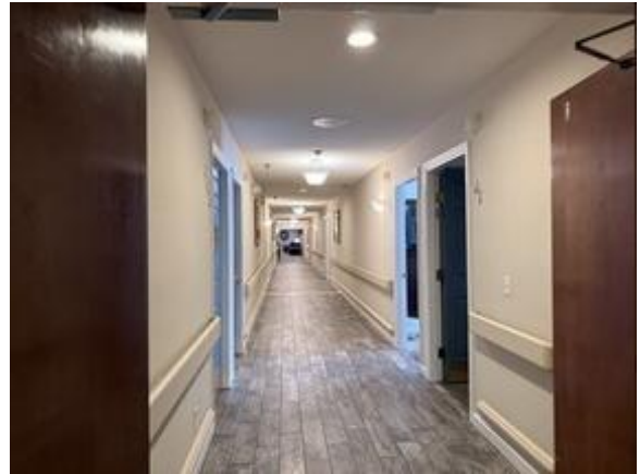
Interior View of Typical Hallway
