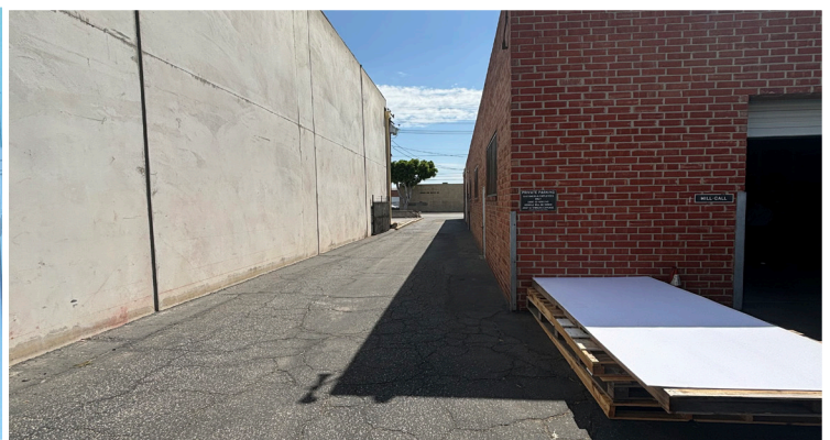
Yard Area-Facing East: Driveway with Access from S Soto Street
