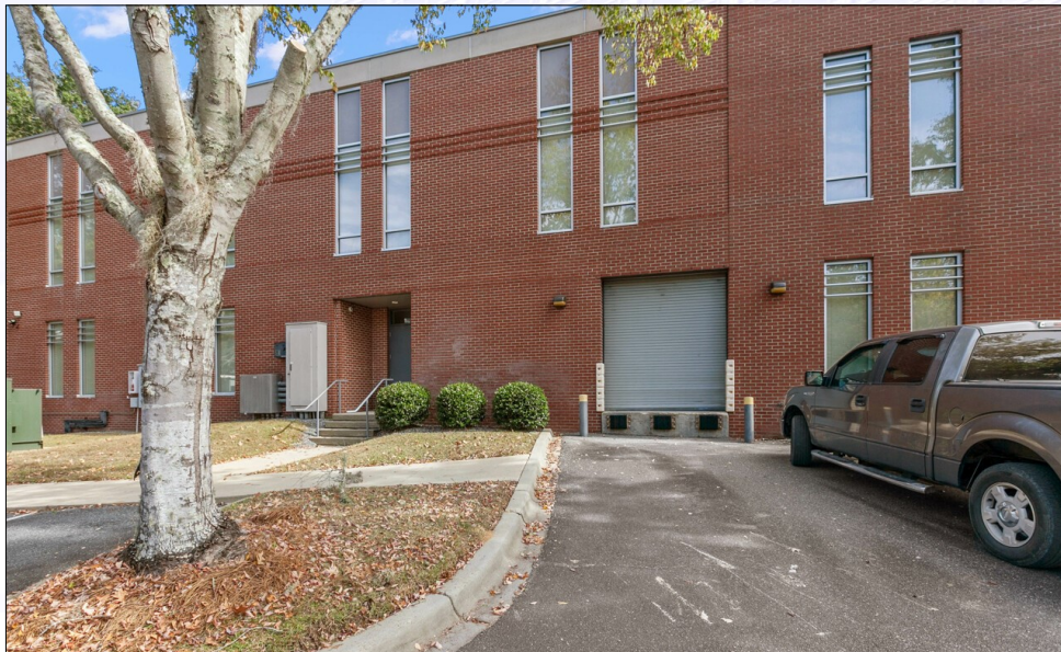
Exterior- Loading Dock
