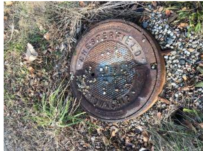
12) Nearby manhole observed due west of pipe observed at Hickey Road.
