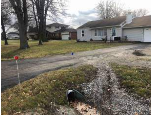
9) View of a roadside pipe east of the wetland area.
