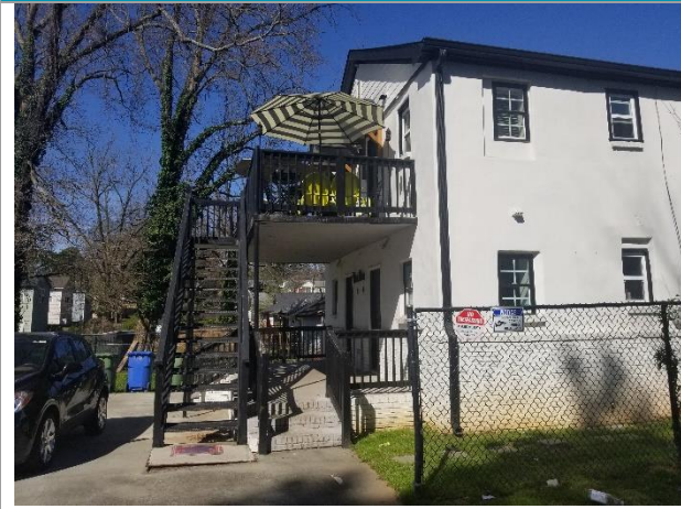
REAR VIEW SHOWING ENTRANCES TO 1BR UNITS AND DECK
