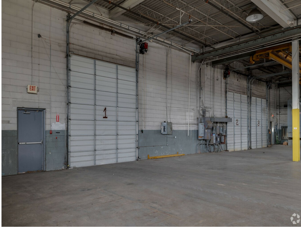
Dock Doors for Efficient Loading Operations
