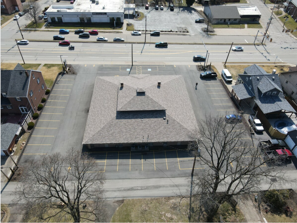
Aerial view from rear
