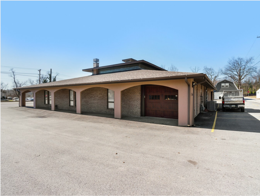
Exterior from right rear corner
