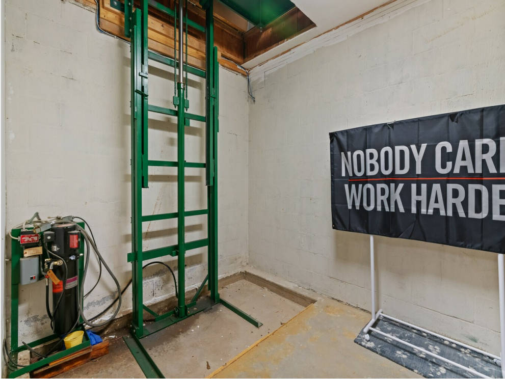
Bottom view of freight elevator from basement
