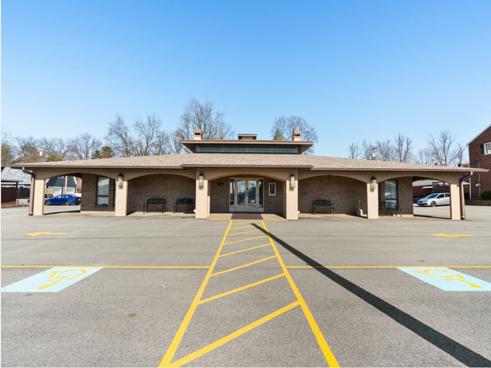
Front view from Freeport Rd
