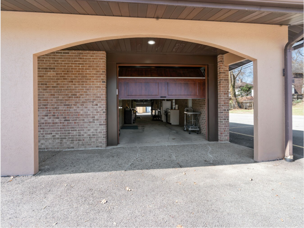
Drive thru garage
