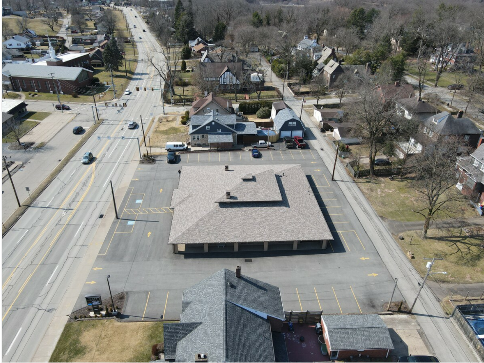
Aerial view from right side
