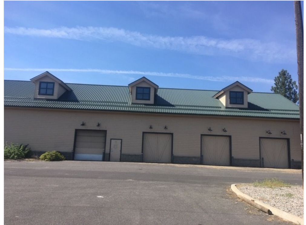
Building N Side
