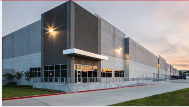
// PARC SOUTHWEST IRVING, TEXAS
