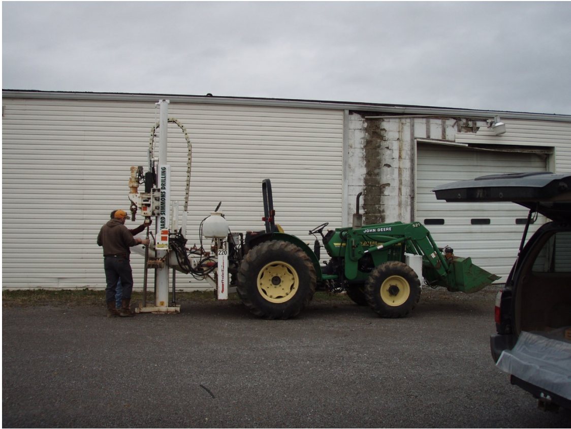
Drilling Boring B1
