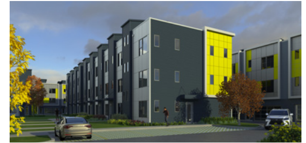
LYRIC CLEVELAND PARK 50 STR UNITS
