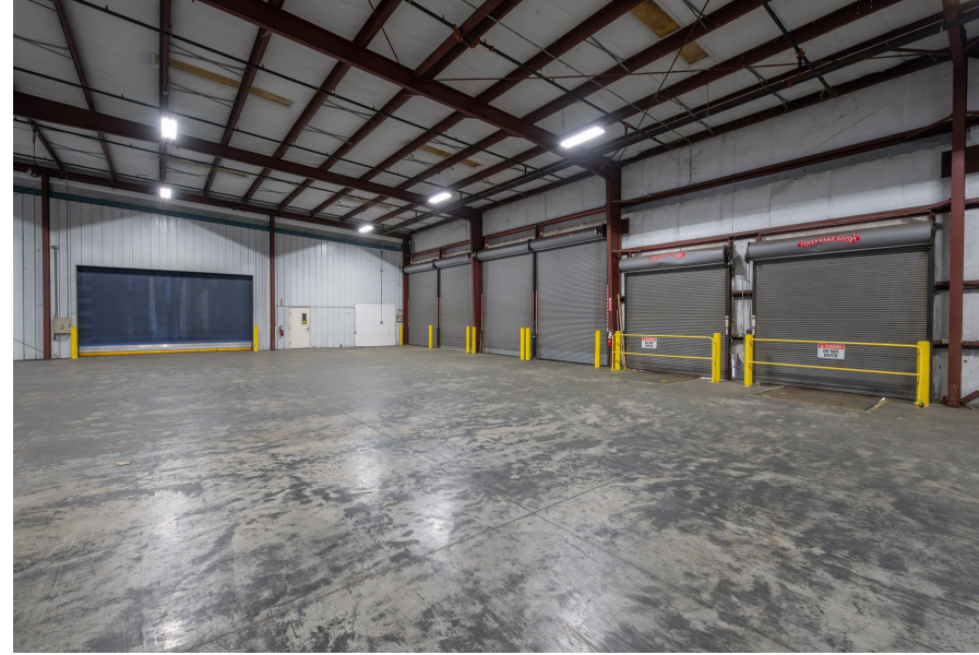
Loading Area | Oversized Grade-Level Doors
