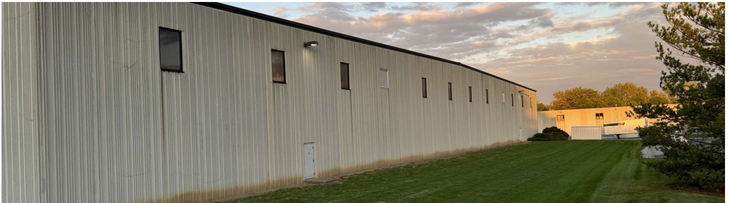
South Side of Building
