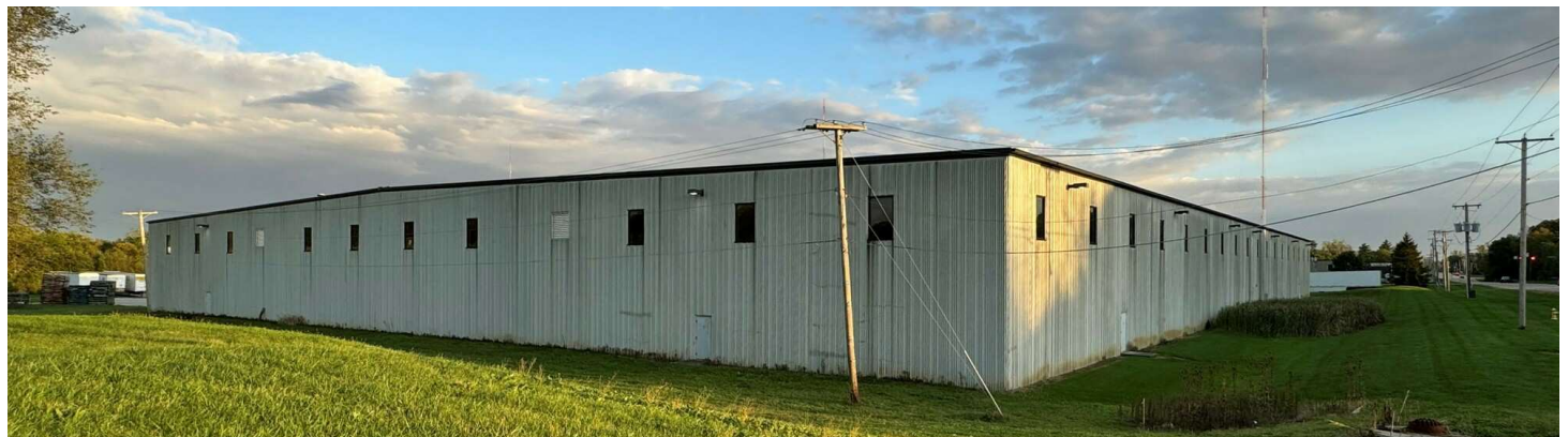
North Side of Building
