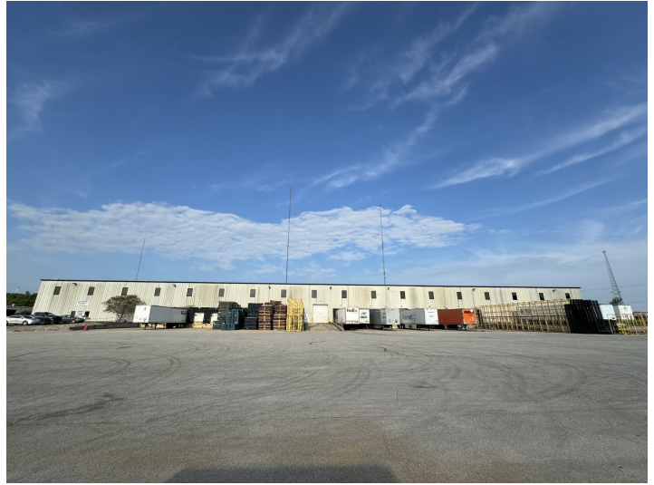
West Side of Building
