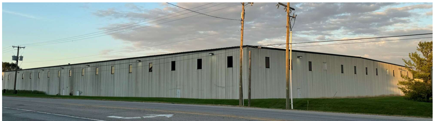
West Side of Building
