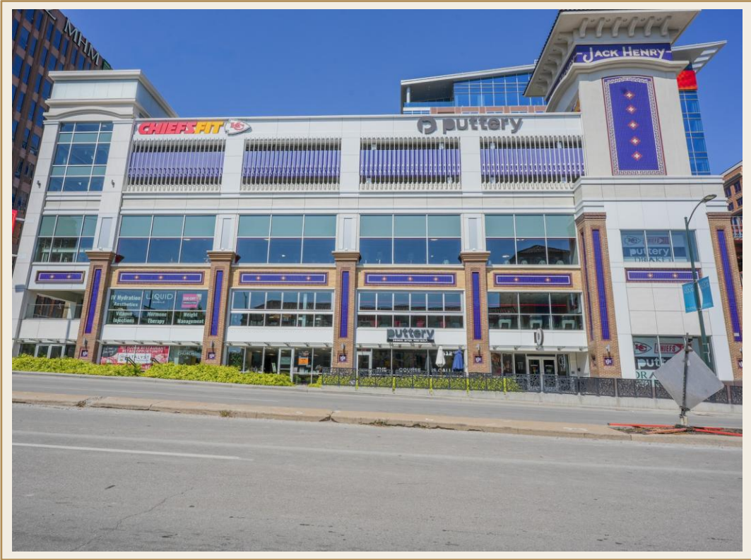
The restored façade on 47th Street
