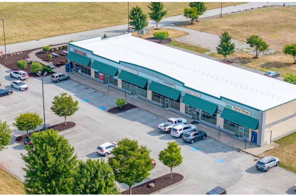
Aerial Facing South
