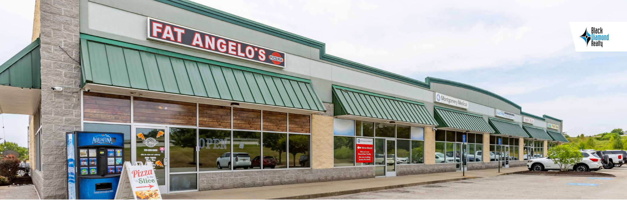
Front of Building
