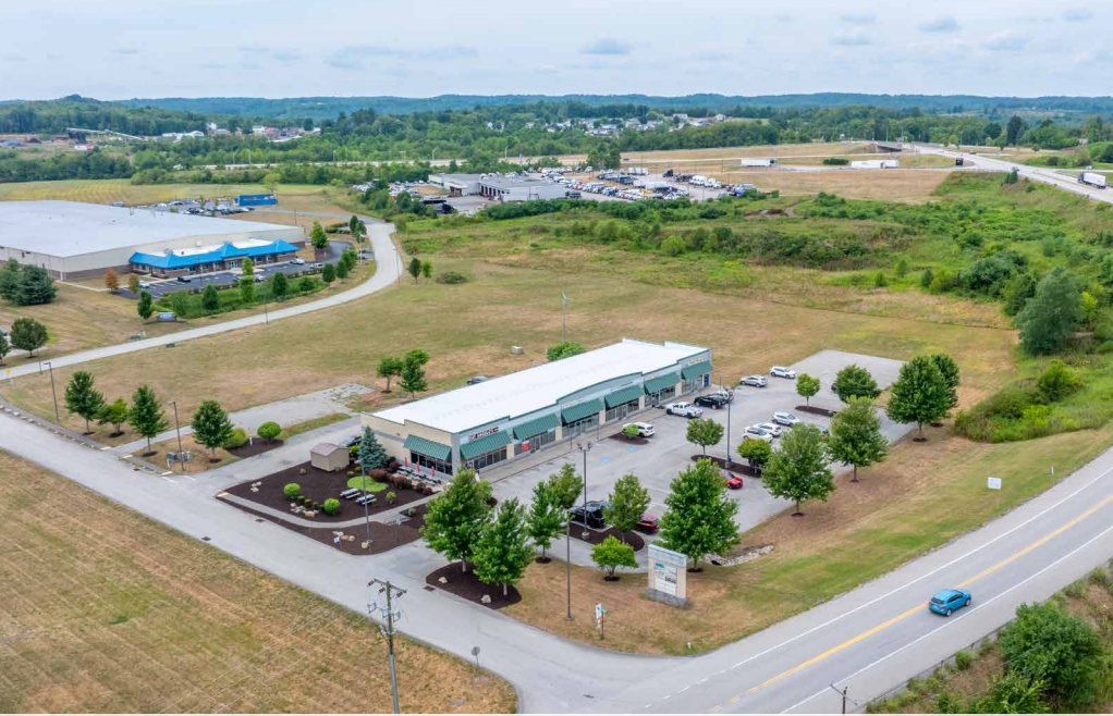
Aerial Facing West
