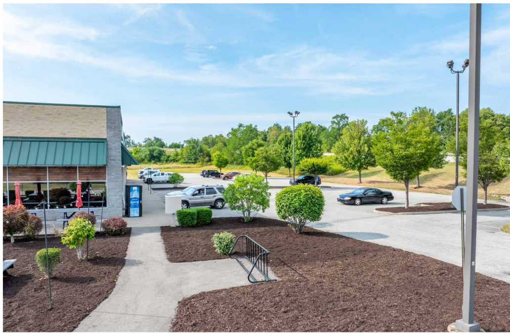
Side of Building
