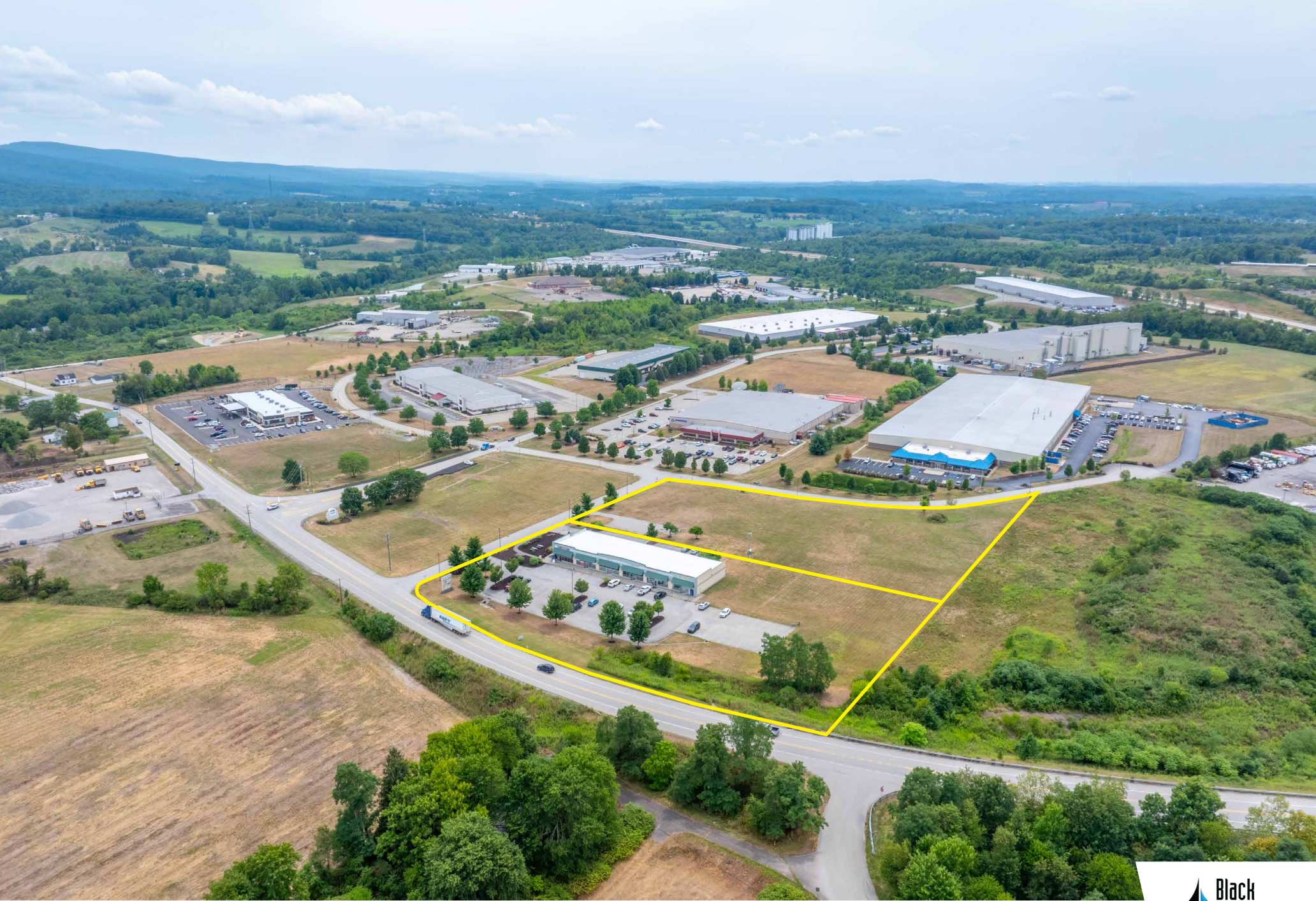
Aerial Facing South
