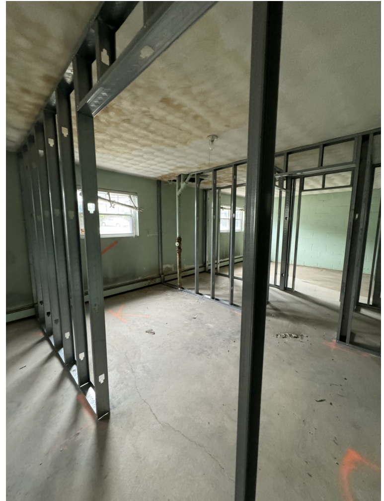
View From Living Room into Kitchen
