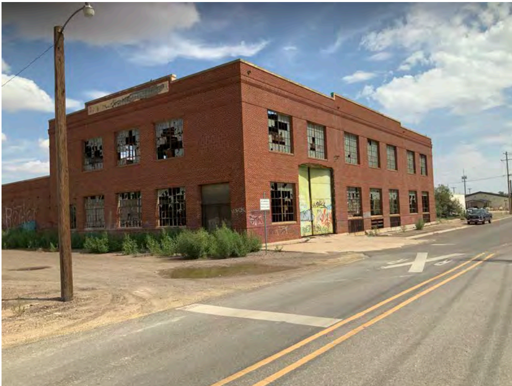
Looking at north and west side of building
