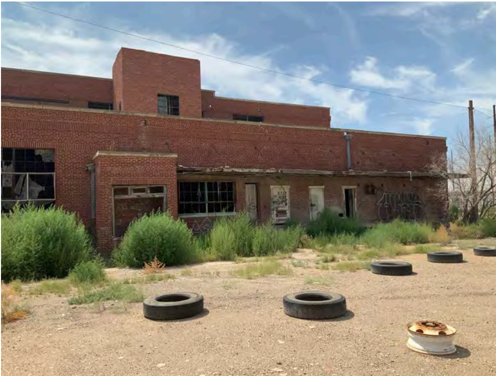
Looking at east side of facility
