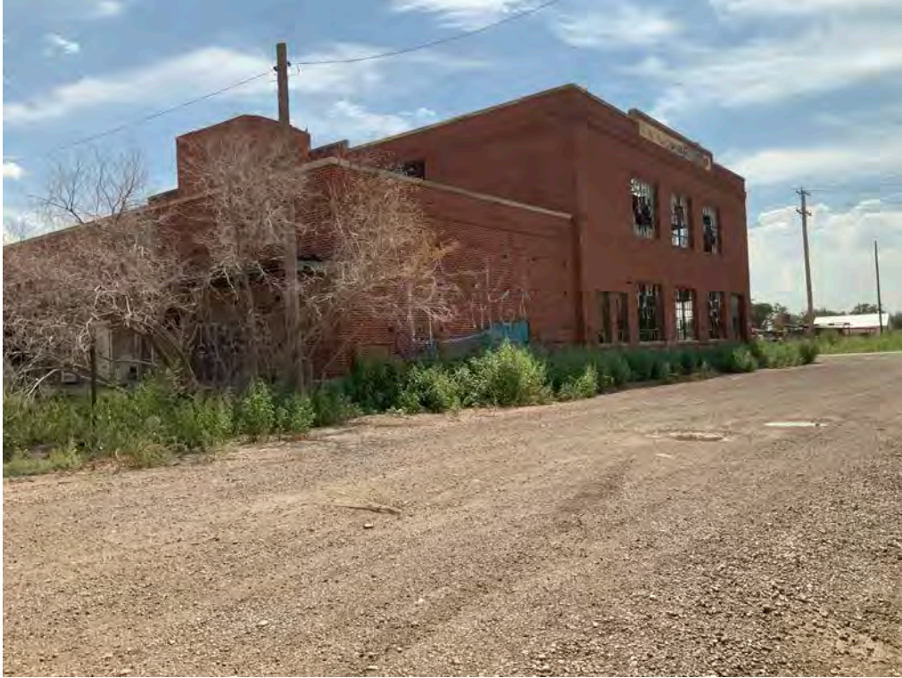
Looking at north side of building
