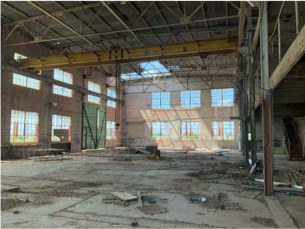
Looking inside main shop room-west side
