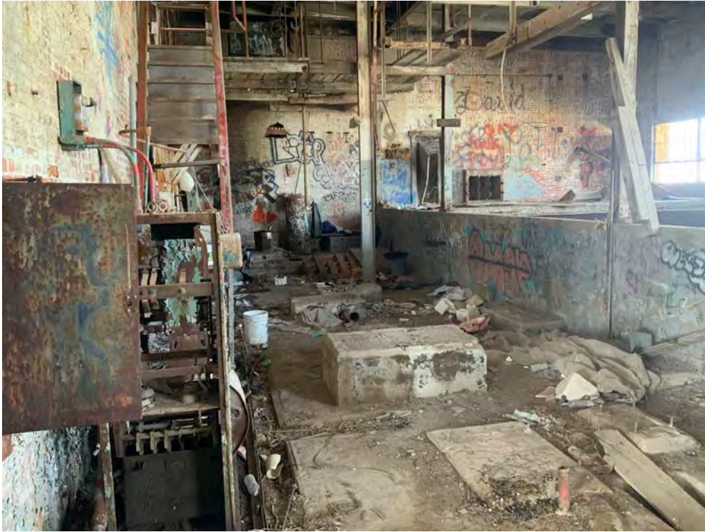
Looking at east shop area
