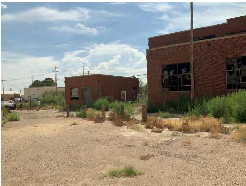
Small building at southeast corner of main building
