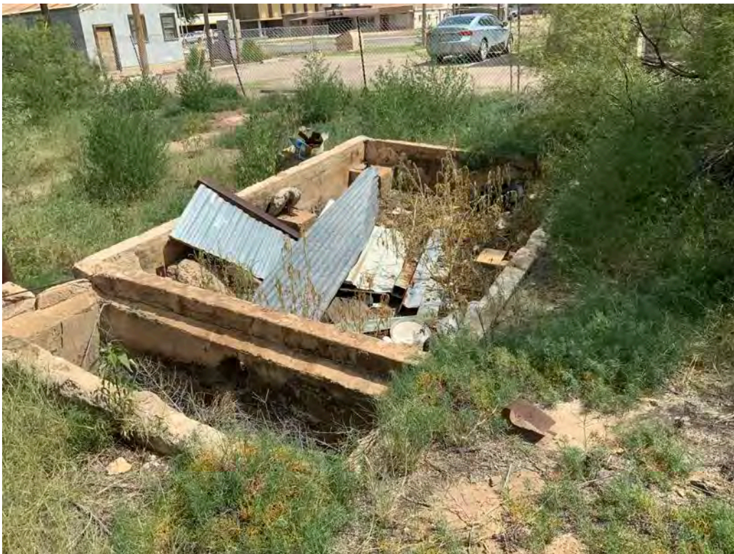
Old water tank in yard area?
