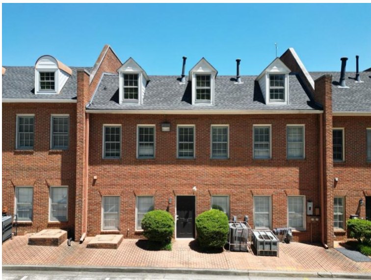
Rear elevation — secondary access and additional parking
