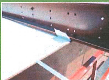
Fabric liner trimmed and sealed to the rafter.
