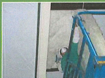
Pull or blow-in JM Formaldehyde-free™ fiber glass insulation between the purlins.
