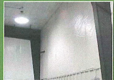
Finished wall and ceiling in manufacturing facility.
