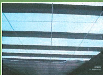
Install the longitudinal and traverse steel strapping to create the strap platform.
